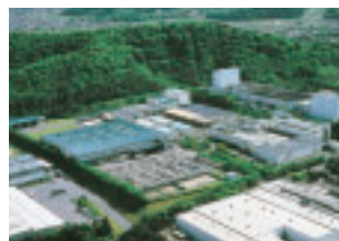
Fukusaki Factory (Hyogo Prefecture)
