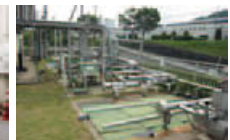
Water treatment facility at the Fukusaki Factory
