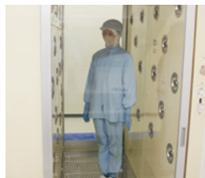
Measures for prevention of contamination by foreign matter (air showers)
